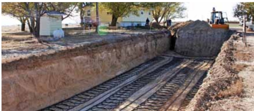
Geothermal heat pumps rely on energy of the ground to move heat into and out of a building, providing winter heating and summer cooling.
