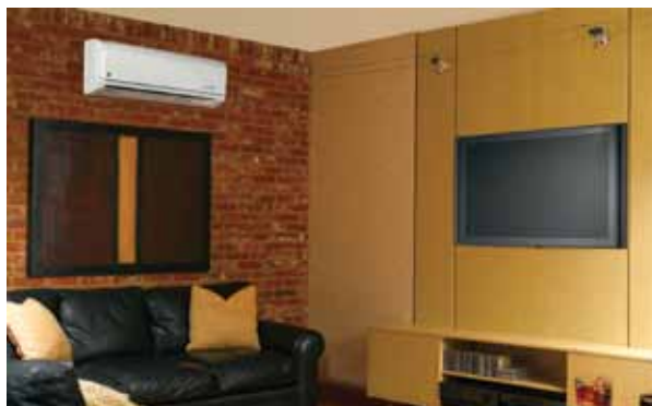
Ductless or “mini-split” heat pumps are ideal for room additions where adding duct work may not be possible.
