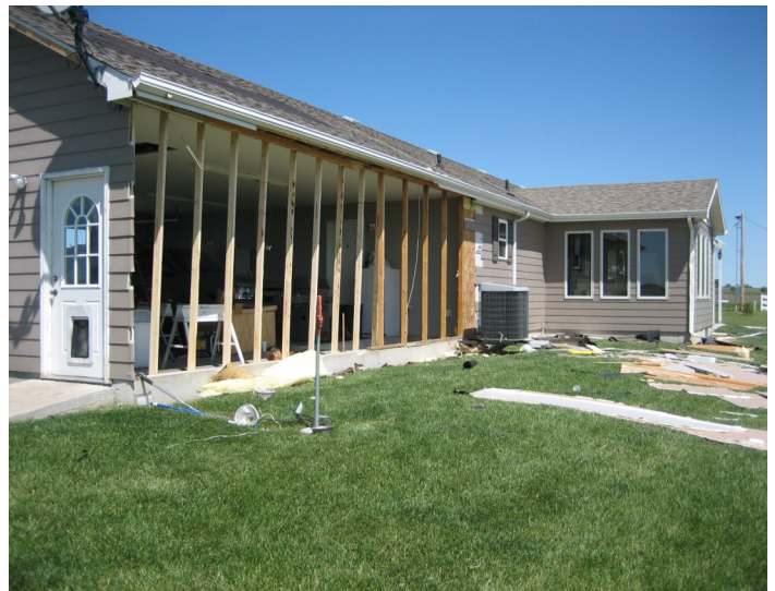
The back wall of a garage near Hope, KS was blown out after the garage door gave way.
